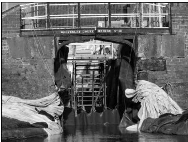
Fabric Dam and Scaffolding Photographs by Ian Cowdale
