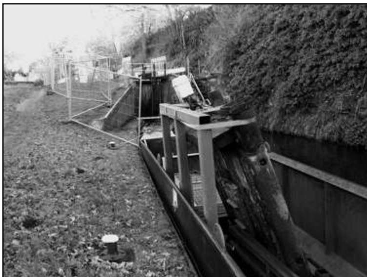
Gate replacement, ladder and brickwork repairs Photographs by Ian Cowdale
