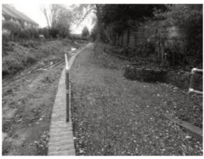
The canal channel along this section has been excavated and the surplus soil material will be moved next year to other parts of the site.
