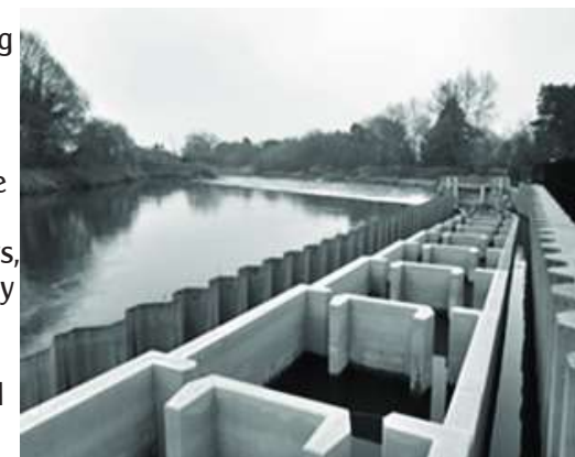
Diglis fish pass after steel pilings cut
