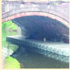
debris was removed from the towpath. Pontoons were collected from Greensforge by road and positioned over the submerged debris to ensure that a clear channel was available.
